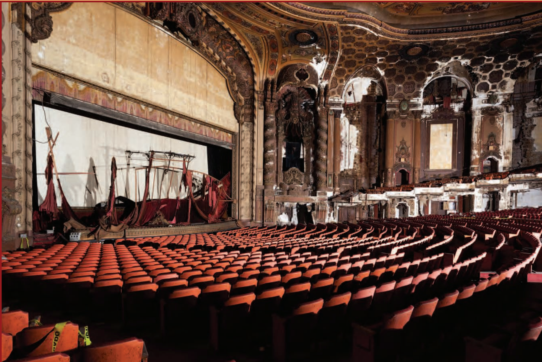
The auditorium, before the renovation. The water damage on the house right wall was especially bad.
