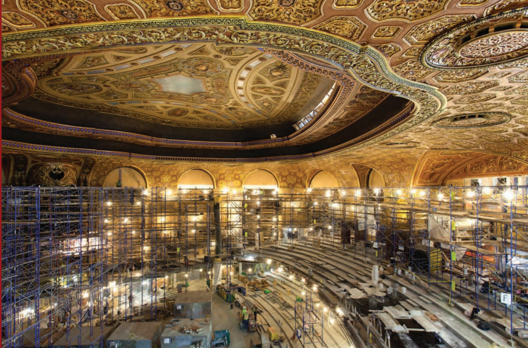
The renovation in progress; EverGreene Architectural Arts restored the decorative walls and ceiling.
