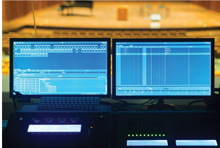
The lighting console allows for additional control.
