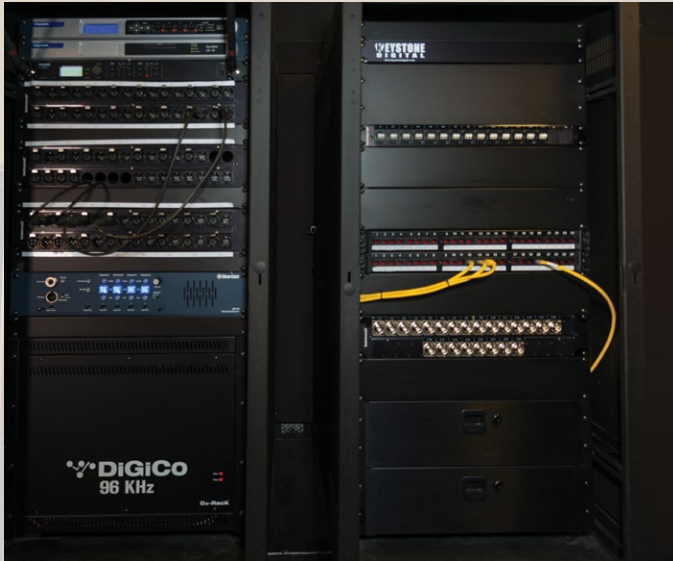
All of the signals from the stage collect at the stage rack. Then lines are distributed between the stage rack and the control booth rack for patching.
