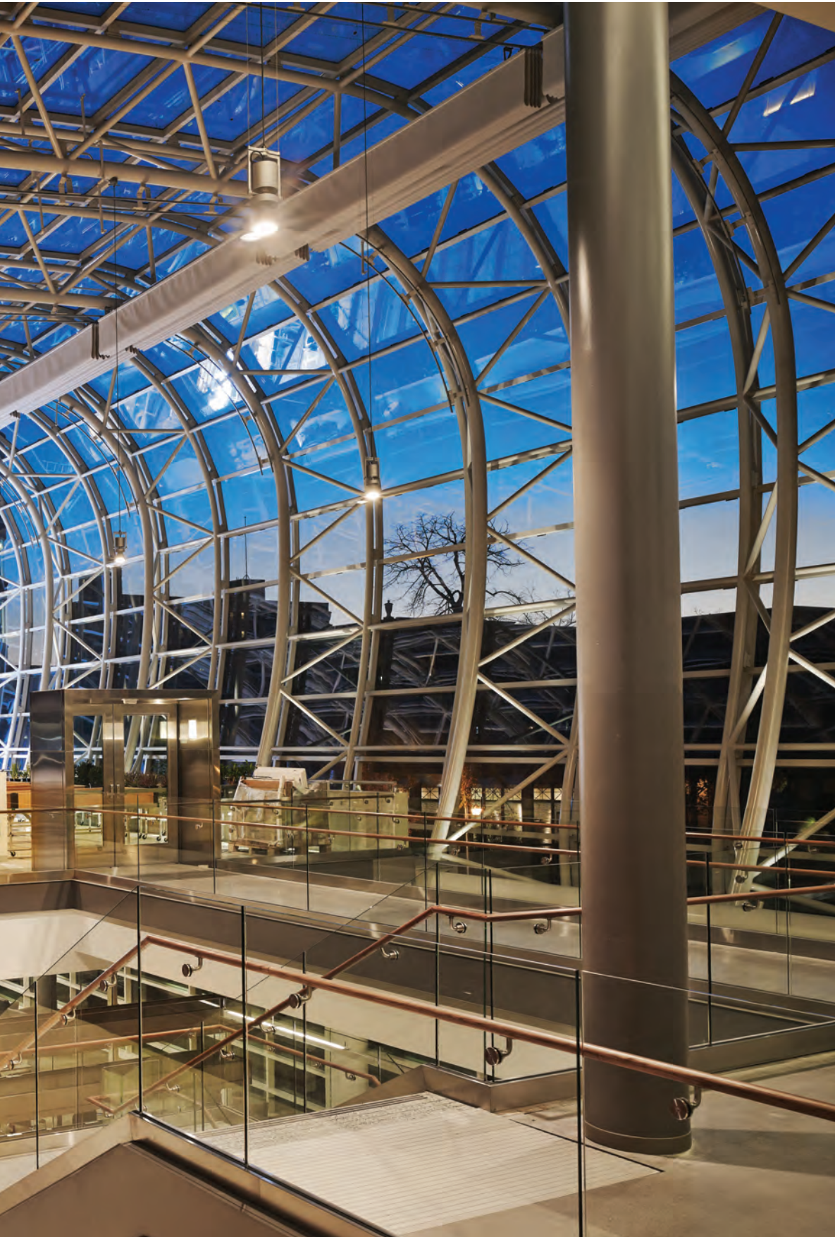
Pendant-mounted CMH downlights designed by architect Renzo Piano light the aquaponics area in the EcoDome, where plants are cultivated without soil.
